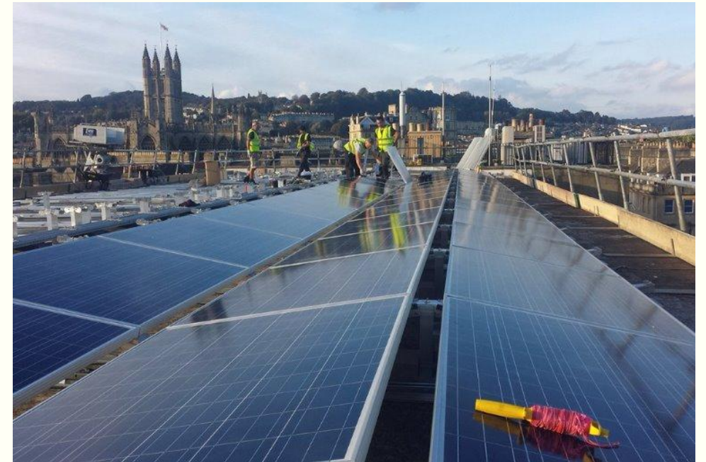
BWCE install of solar PV at Council office Lewis House
