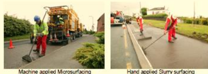
Machine applied Microsurfacing
