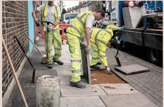
Nu-phalt teams in operation on EM Highway Service Enfield contract
