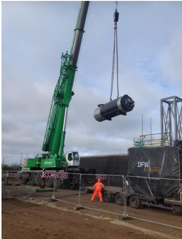
Huntingdon Crematorium first of two DFW electric cremators being installed
