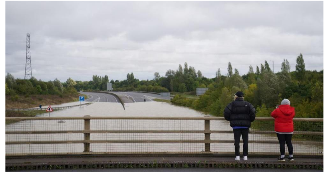
National Highways expects part of the A421 main road in Bedfordshire to remain closed on Tuesday after it was submerged by flooding
