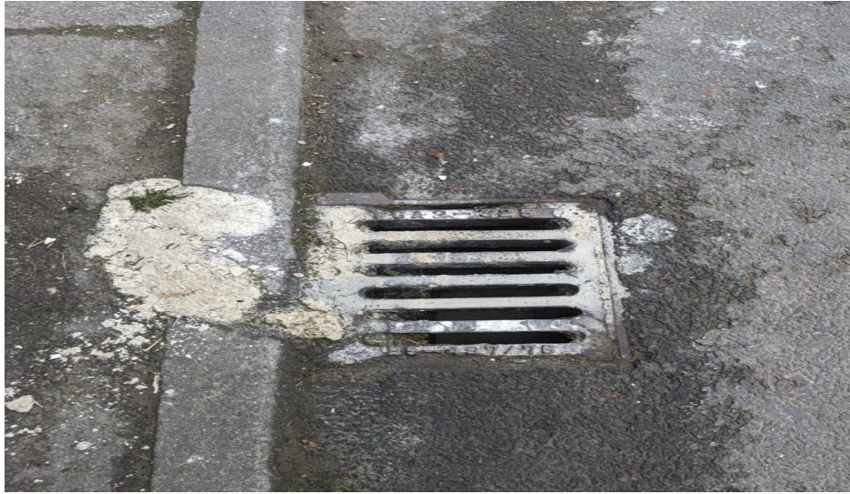
Concrete into gullies
