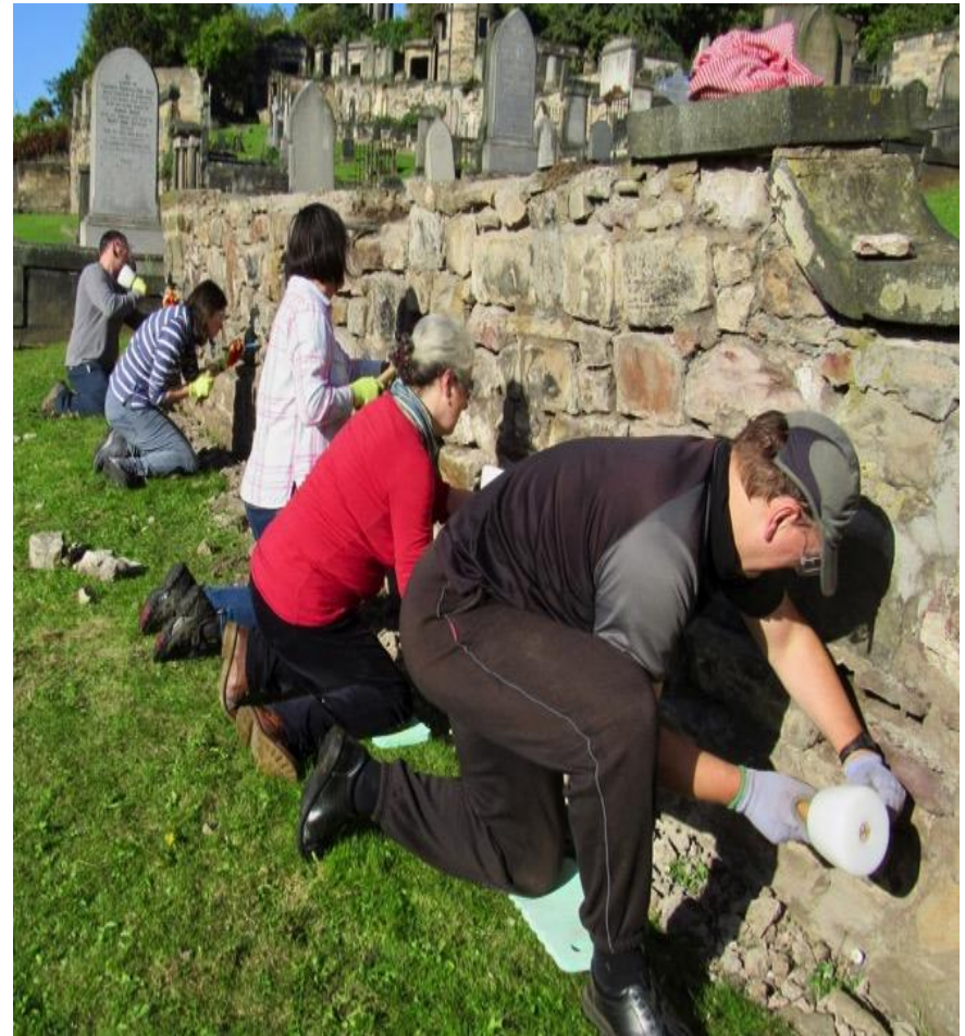
Volunteer workshop repointing terrace wall with lime mortar
