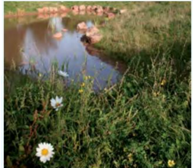
Marissal Road attenuation pond
