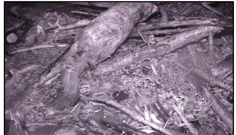
Debris Screen 9th Feb
