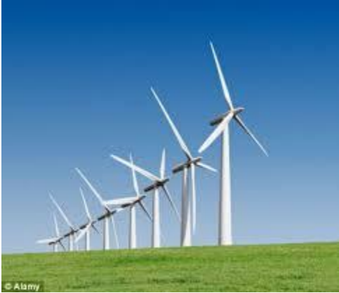
Third party generator
