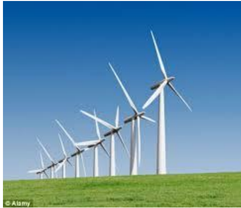
Third party generator
