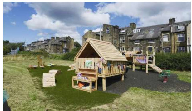
Primary school play equipment installed by the Better Place project.
