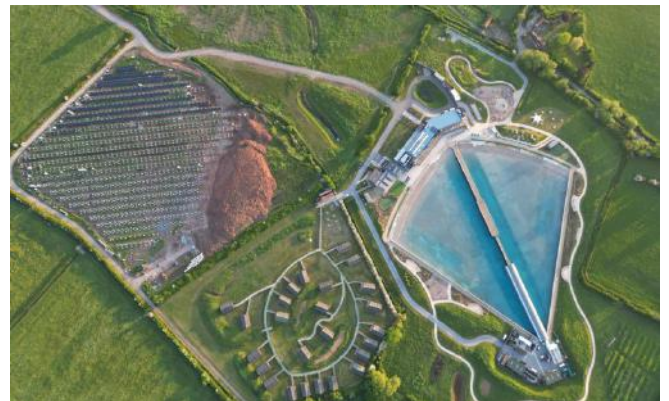
'The Wave' inland surfing lagoon in South Gloucestershire, powered by a solar 'Smartflower.'
