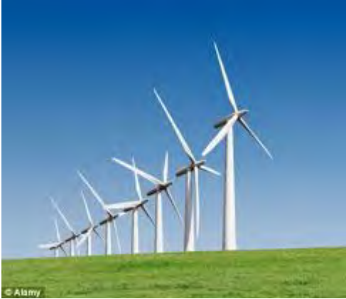
Third party generator
