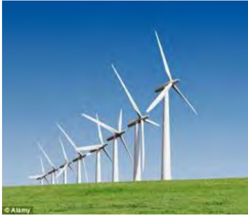
Third party generator
