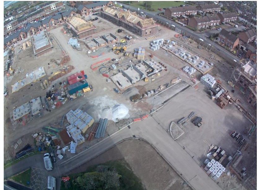
Progress to date on site
