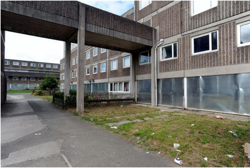
View of the existing maisonettes pre-demolition
