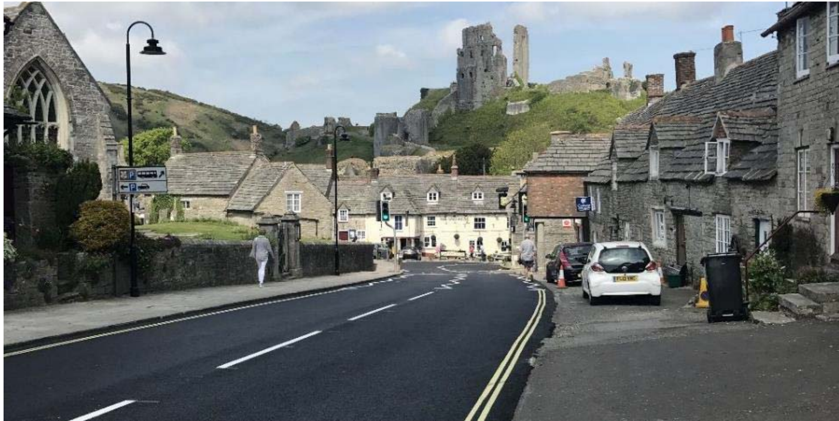
Corfe Castle Resurfacing
