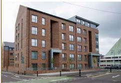
Each phase of the Anderston masterplan has been delivered using off-site Modern Methods of Construction with CCG OSM designing and manufacturing the enhanced closed panel timber solutions that were installed upon 2 storeys of traditional brickwork. The housing was designed using the Fabric First approach and achieve a Silver Eco Rating, an important factor in reducing fuel costs to tenants.
