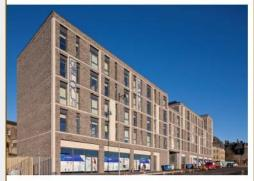
As an extension of the historical context of the City, the building is formed by the use of black and grey brick for the exterior façade and a soft grey render finish applied to the south elevation. Facing Station Road, Goosecroft also plays homage to the artistic merits of Stirling by including five, contemporary stone panels, commissioned in partnership with Creative Stirling.
