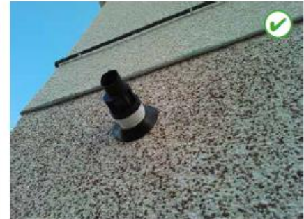
Figure 37: sealed penetration (good practice)
