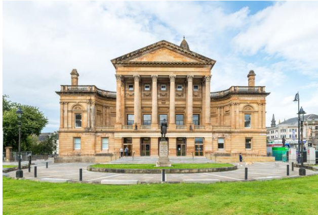
Paisley Townhall Refurbishment - £22m investment
