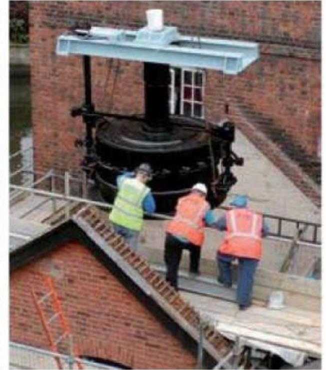
Figure 54: The Town Mill in Guildford showing the single storey Toll House and (right) the 35kW hydro turbine during installation
