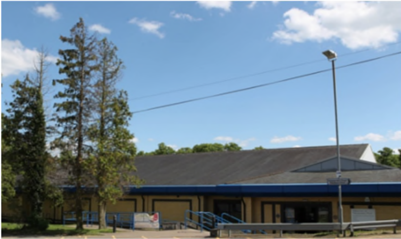
Existing swimming pool
