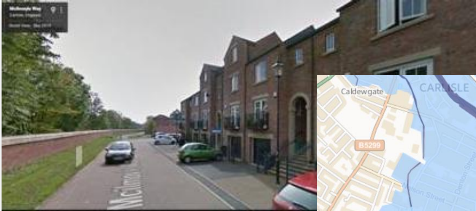
Mcilmoyle Way, Carlisle – flood wall, raised floor levels, ground floor used for parking
