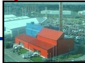
The Heat Station
