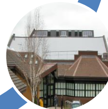
Solar PV on Commercial Buildings
