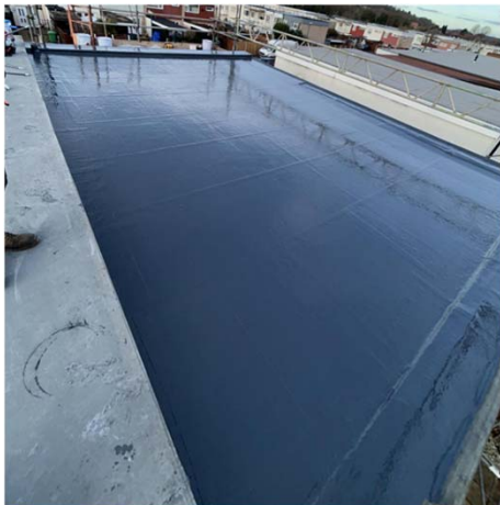
Flat Roof Insulation
