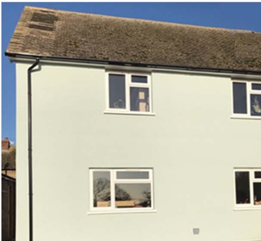
External Wall Insulation
