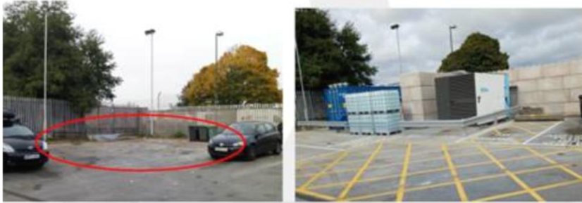
Mobile Refuelling Station Site Marsh Road, Alperton
