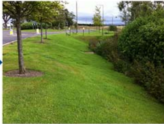
Linear wetland → long swale → sediment basin
