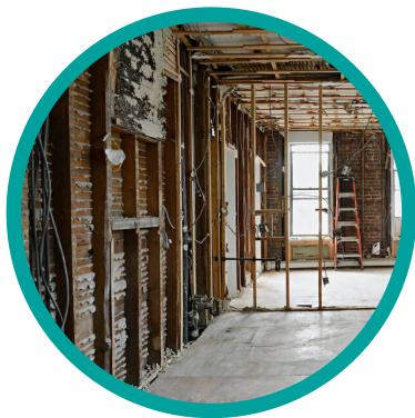
Major property renovations
