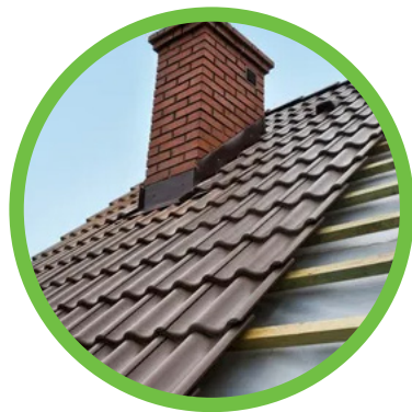
Roof or thatch replacements
