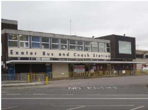
Bus Station Regeneration
