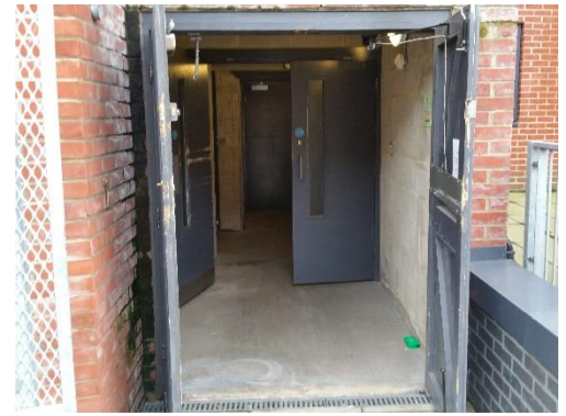
(Fig 2) Entrance to underground storage area
