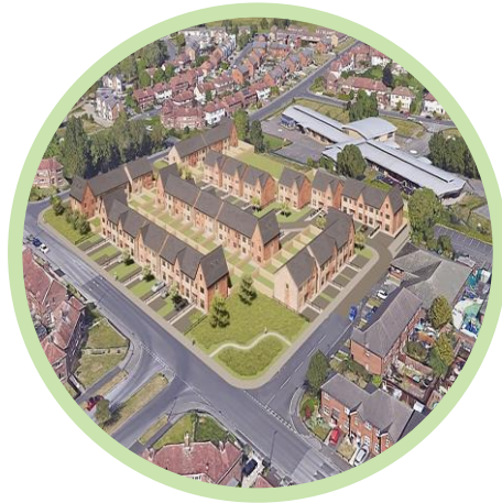
30 new Council homes with air source heat pumps, solar power and battery storage
