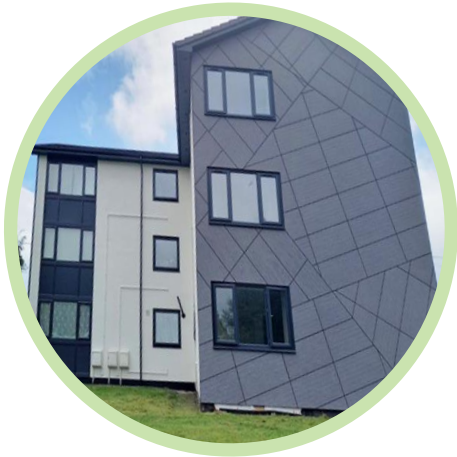
Garstang Road West Flats retrofit programme
