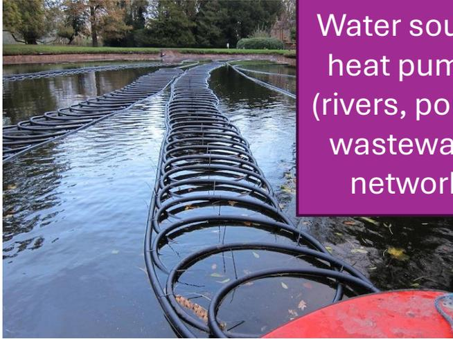
Water source heat pumps (rivers, ponds, wastewater network)
