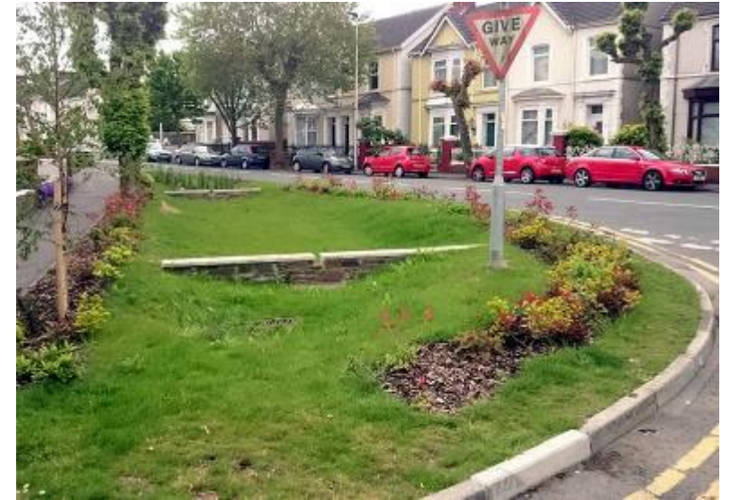
Vegetated swales with flow controls
