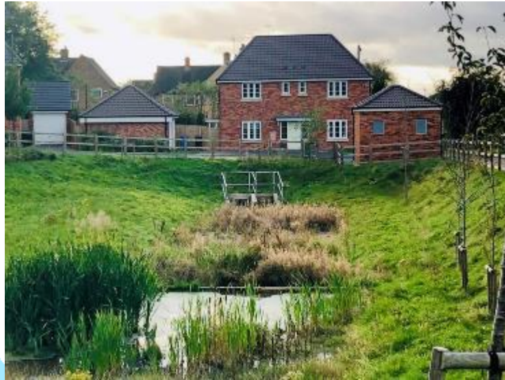
Constructed wetlands and attenuation basins
