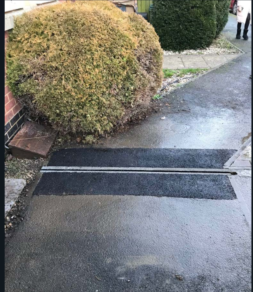
The contrast between new and old tarmac will fade over time
