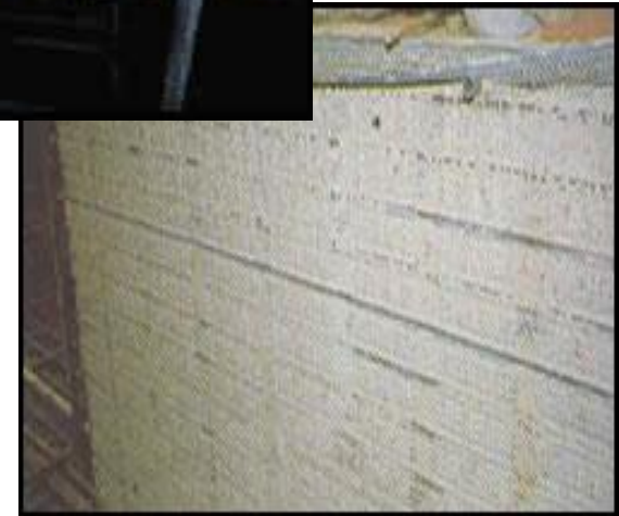
Formwork to eliminate scabbling
