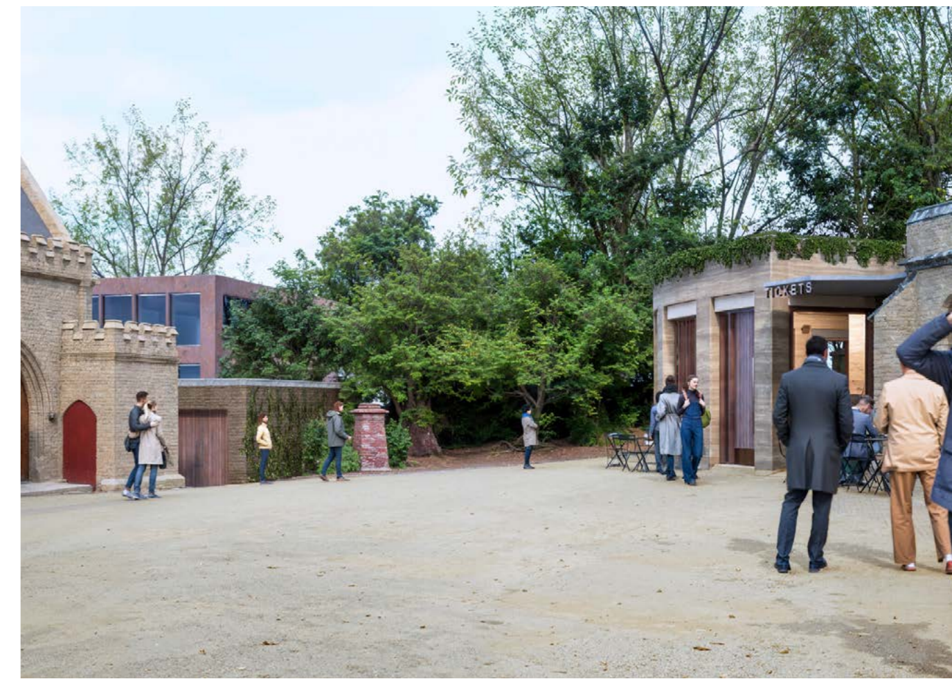
Courtyard Utility Block
