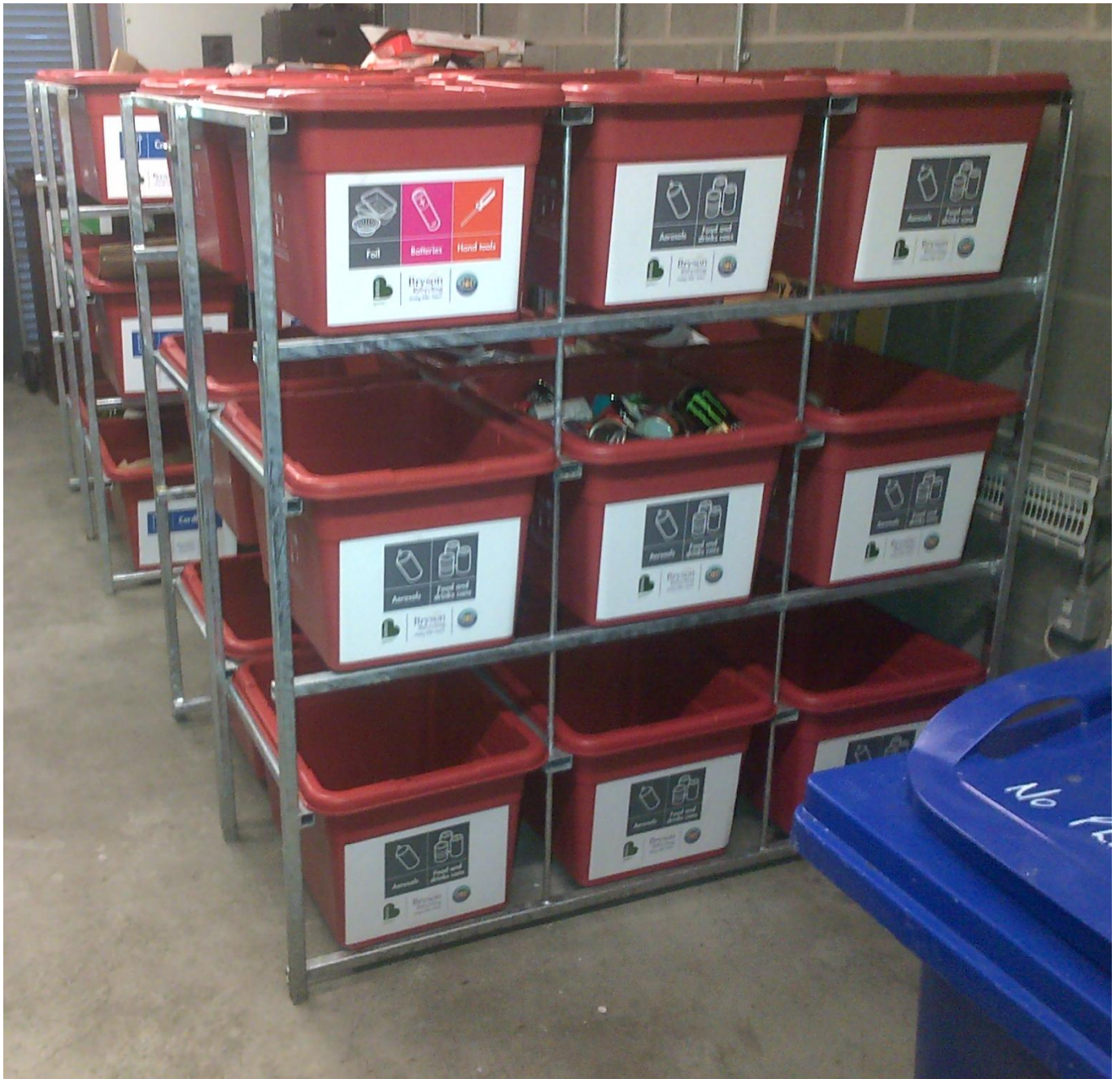
3-tier stand. Overall height reduced by not having lids on each tier – therefore only suitable for indoor locations.
