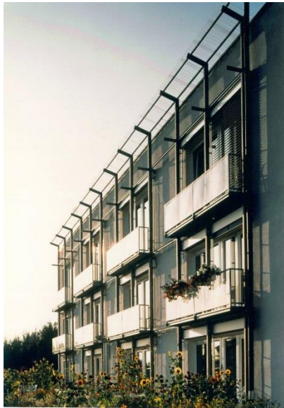
The world's first Passivhaus is built in Darmstadt
