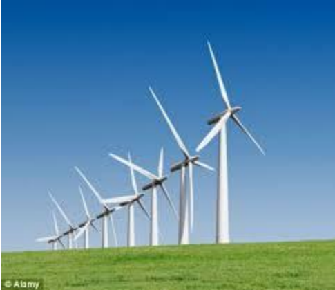
Third party generator
