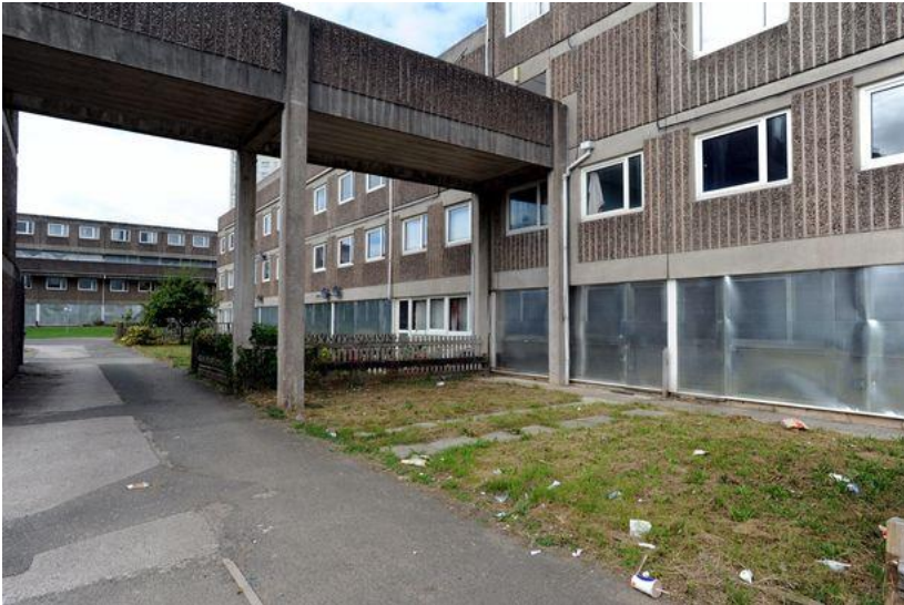
View of the existing maisonettes pre-demolition
