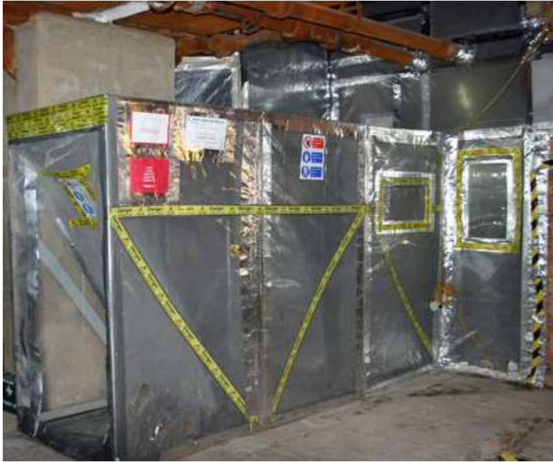
Asbestos enclosure with three stage airlock/baglock
