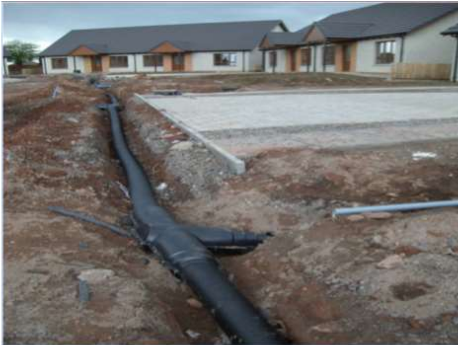
Figure 10: District heating pipes
