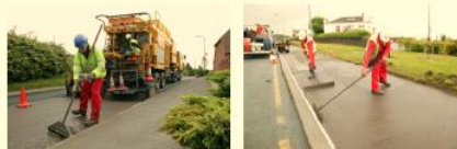
Machine applied Microsurfacing
