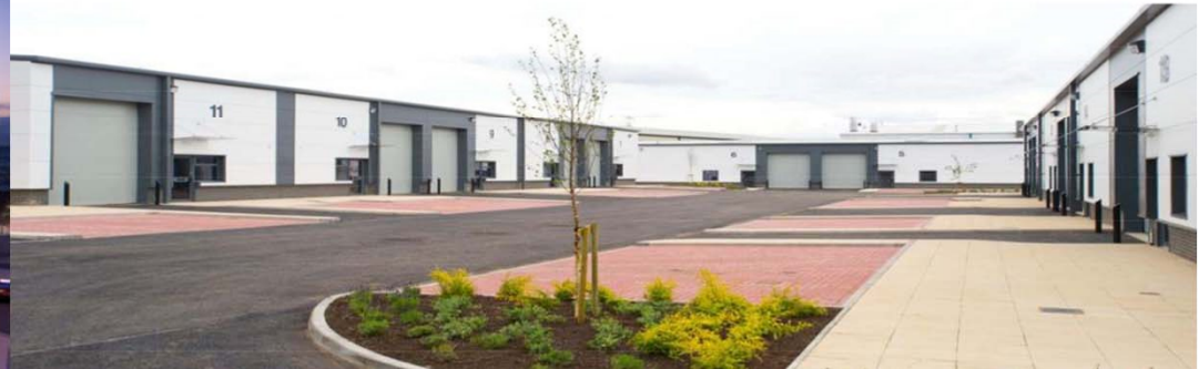
West Chirton Industrial Estate, North Shields
