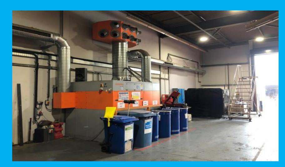
Kemper mobile LEV unit for close quarter working in conjunction with full PPE, E.G. Fire proof coveralls, aprons, gauntlets, air filtered breathing apparatus etc.
