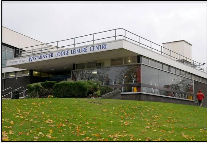
Replacement of old centre built 1971
