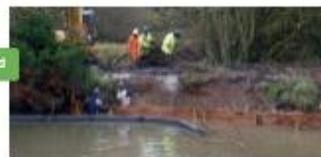
People enjoy using the many paths of the reserve. This picture shows works to strengthen the river bank using coir rolls and a dead tree anchored to the bank, diverting the river away from this bank. The path has also been realigned.
