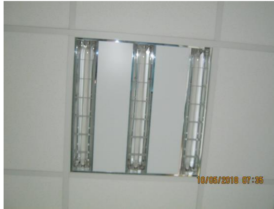
2ft T5 Lighting = low energy saving potential
