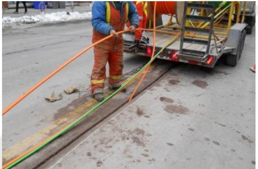
The method of cutting/excavation used for micro trenching can have a significant impact on the ability to achieve an effective reinstatement. The greatest threat to effective reinstatement is the presence of excess moisture. For this reason, a dry cutting process using a vacuum recovery system for the arisings is preferred.
