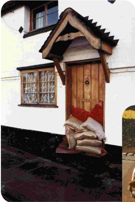
Sandbags and plastic sheet
