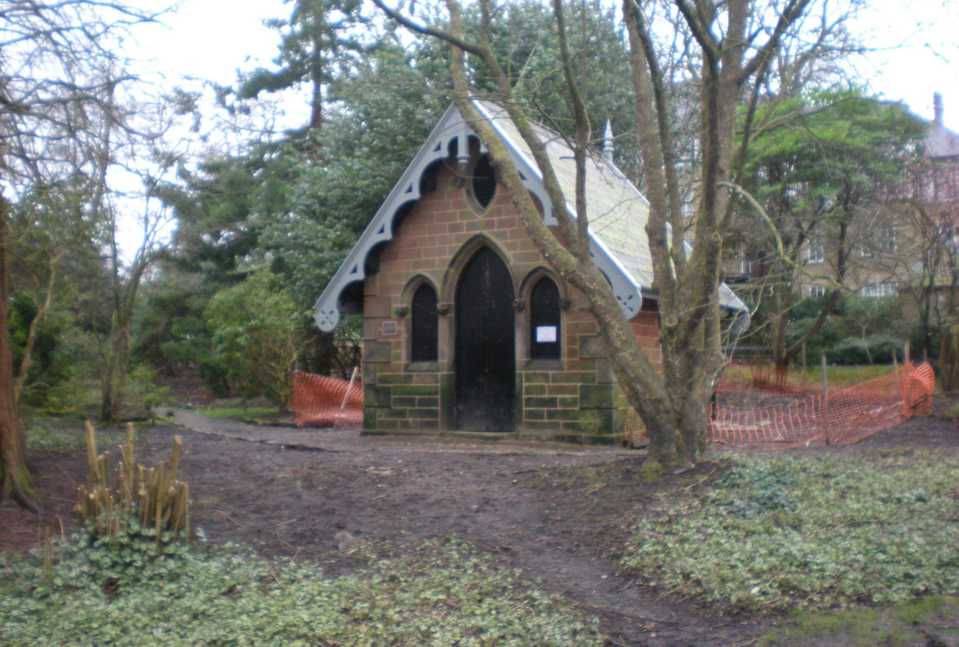
During the renovation
