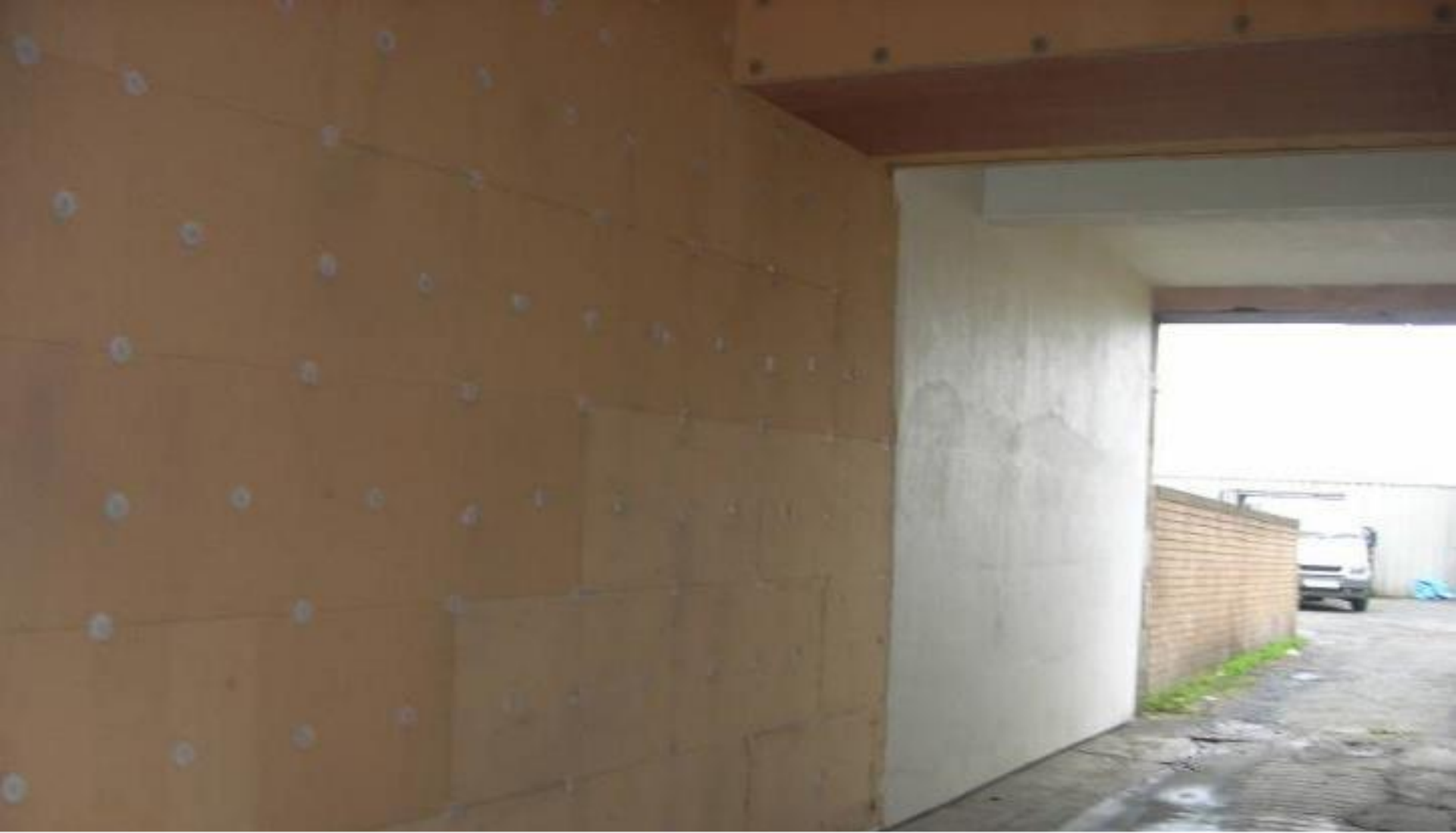
Wood fiber insulation, Glasgow, fixed with thermally decoupled expansion fasteners directly to masonry
